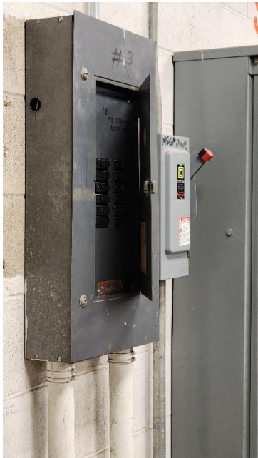
Photo 7: Hangar LP-B #3 Panel
