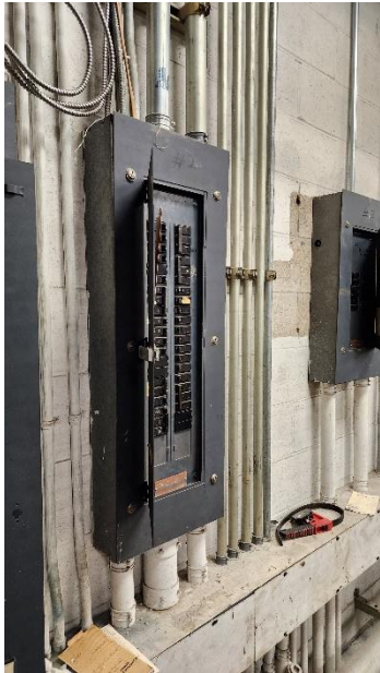
Photo 5: Hangar LP-B #2 Panel
